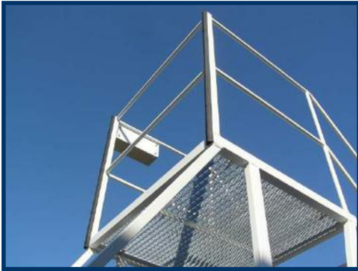
Top platform with toolbox on the left handrail.
