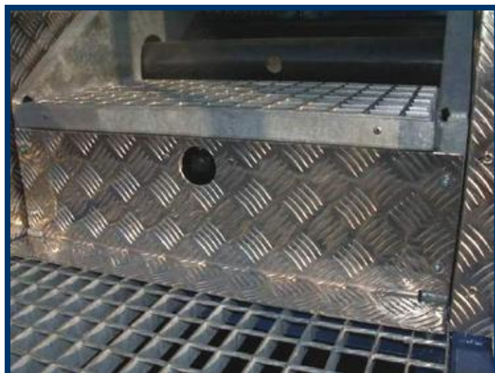
The top wall is covered with an aluminium sheet with slip-resistant treatment.
