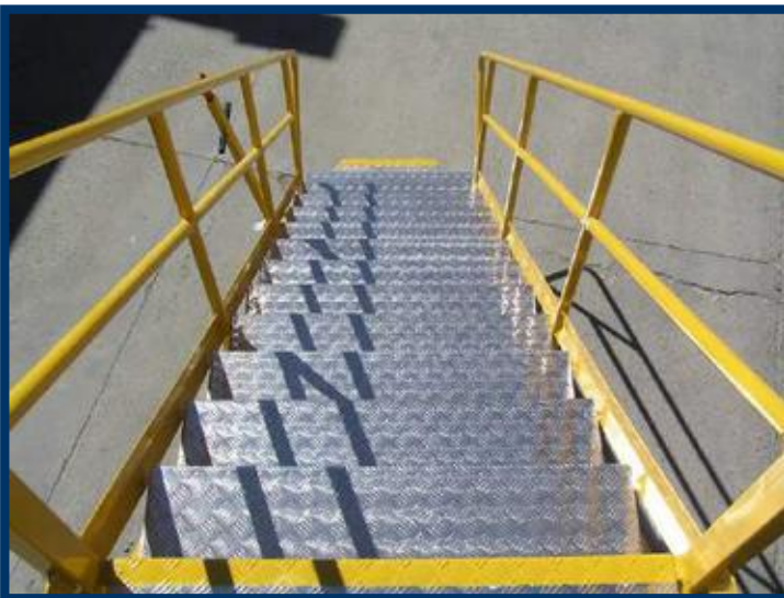
Steps and platform covered with aluminium antiskid sheet.
